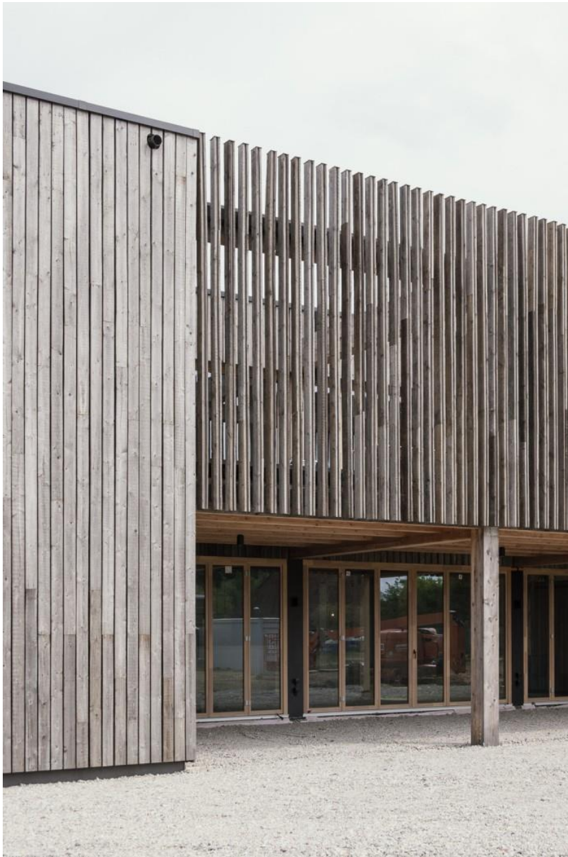
© Jasmien Smets – image 3: reused wooden facade
