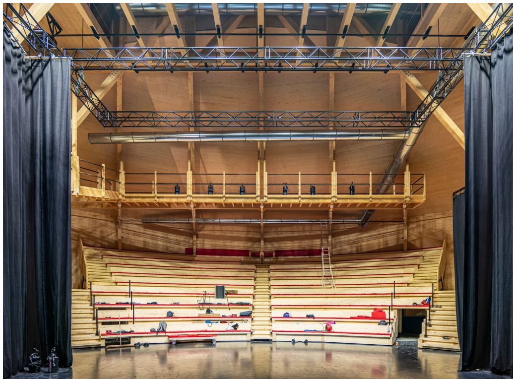
Image 3 : Photo gradin - © Atelier d'architecture Meunier-Westrade
