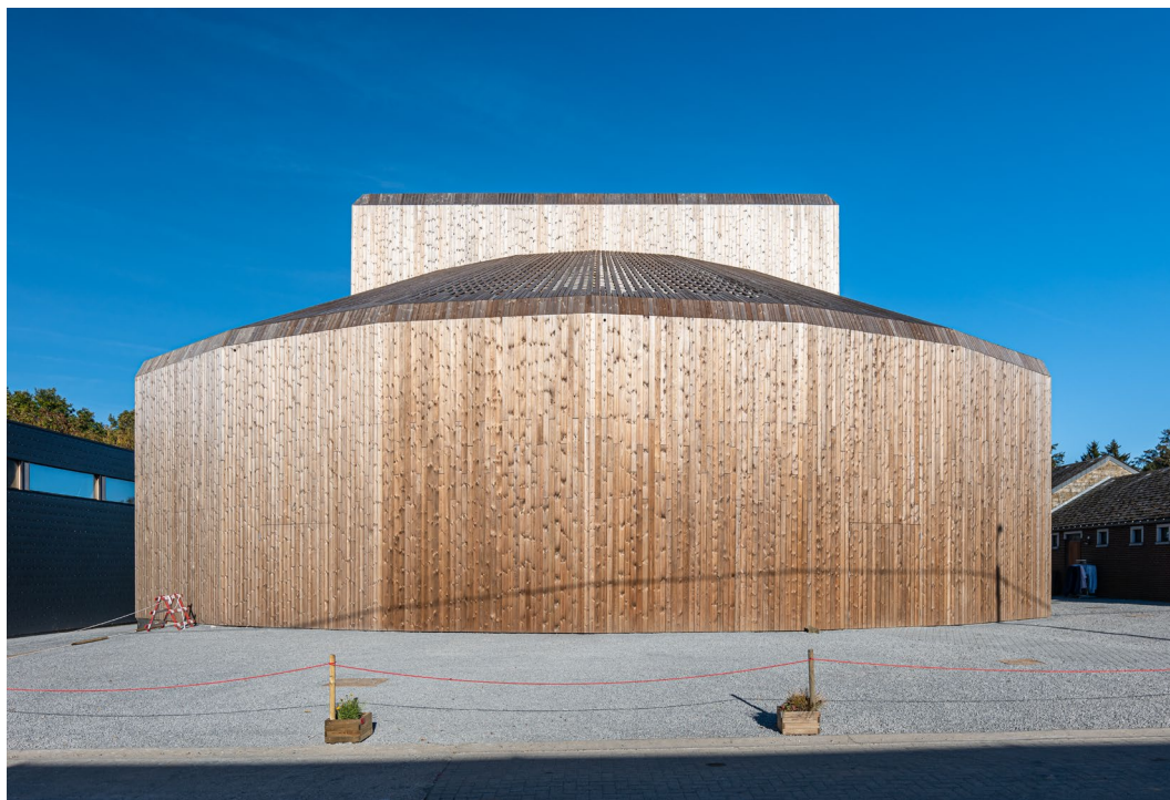
Image 4 : Photo façade - © Atelier d'architecture Meunier-Westrade
